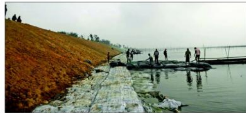
Sand-filled geobags being used for protection of the Brahmaputra riverbank at Hekru in Guwahati, on Saturday - IRI Photos
